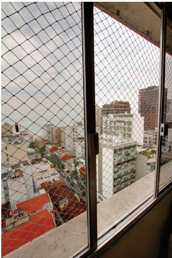
Figure 12. Right image with a tape to set the NPP
